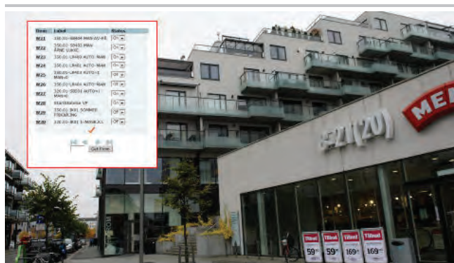
HOT OR COLD?: Dagbladet was able to control the heating in a whole block of apartment buildings here in the city Drammen.
